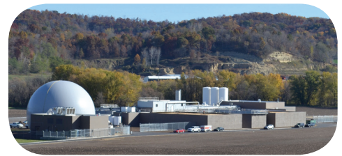
Richland Center Renewable Energy, LLC (RCRE) digester.
