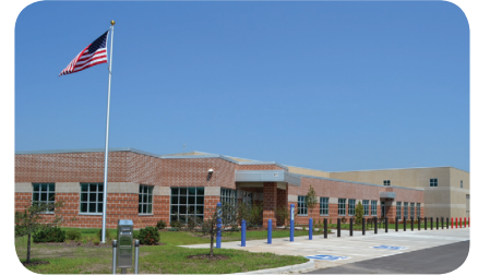
Plymouth Utilities' Operations Center.
